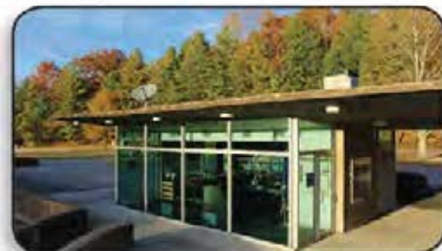
Norris Dam Visitor Center
